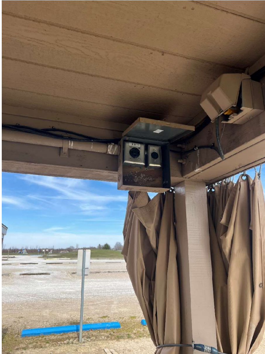
This is also located at the “South Location”. These are 30amp plugs. Zoom in on the image to see it better.
